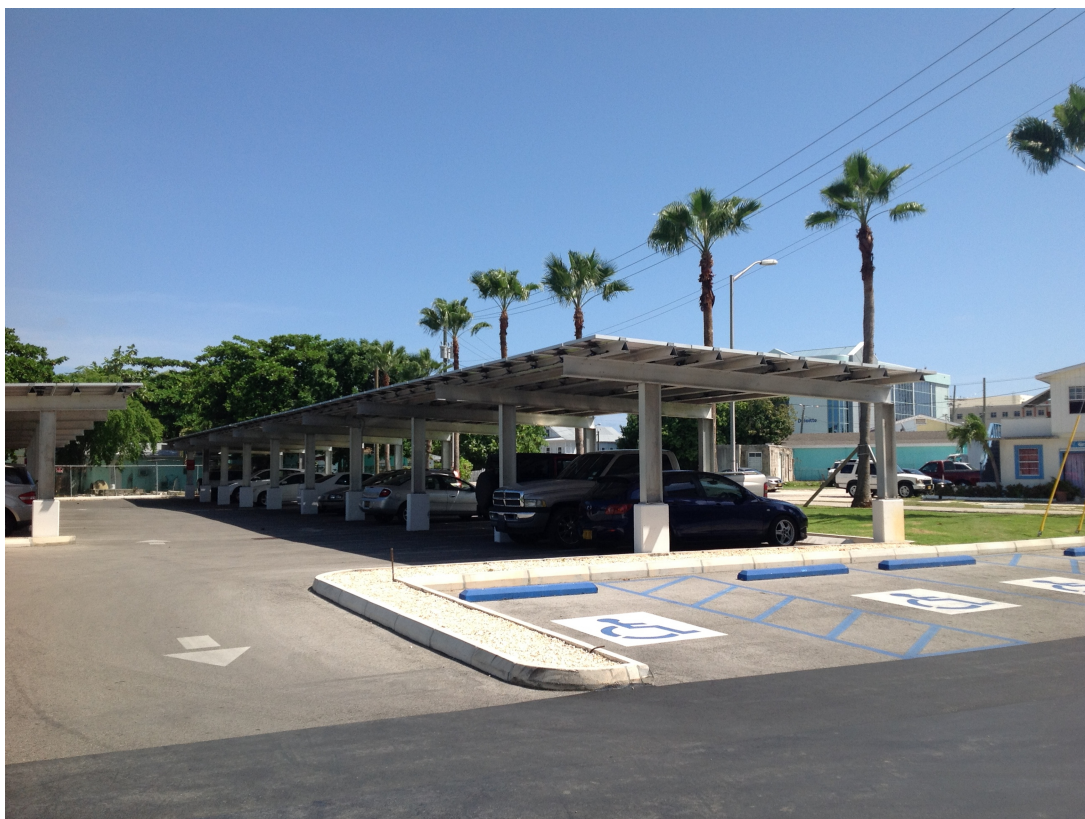
Photo: Engineered car park on Grand Cayman utilizing solar photovoltaic (PV) panels to produce clean energy for export into CUC's T&D system.
