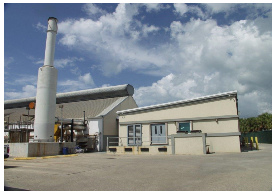
Photo: Control room at CUC's North Sound Plant on Grand Cayman.
