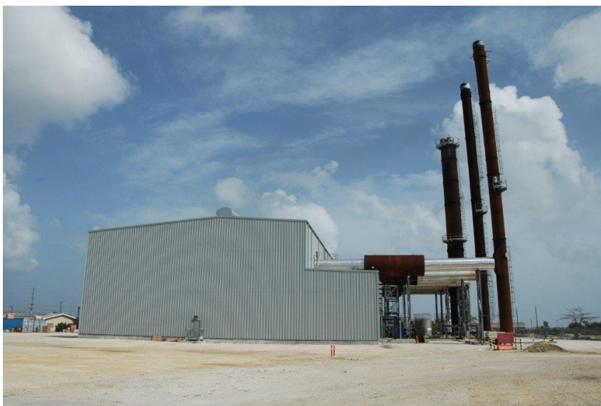
Photo: Engine Room 5 at CUC's North Sound Plant on Grand Cayman. The engine room houses 68.75 megawatts (MW) of diesel generation.
